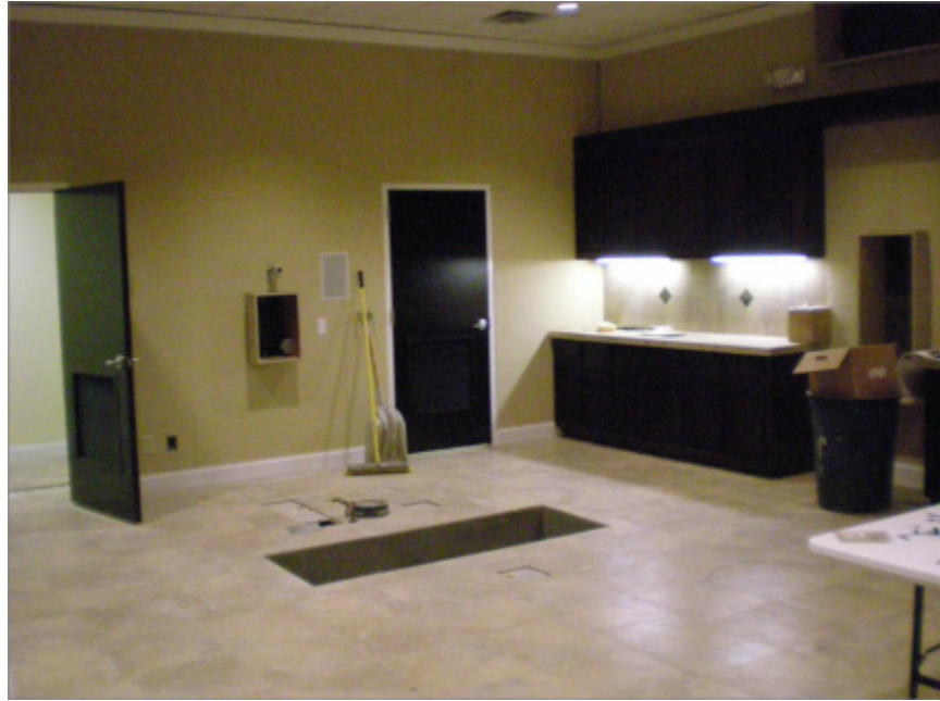
Figure 4-2: Treatment Vault showing gantry pit.
