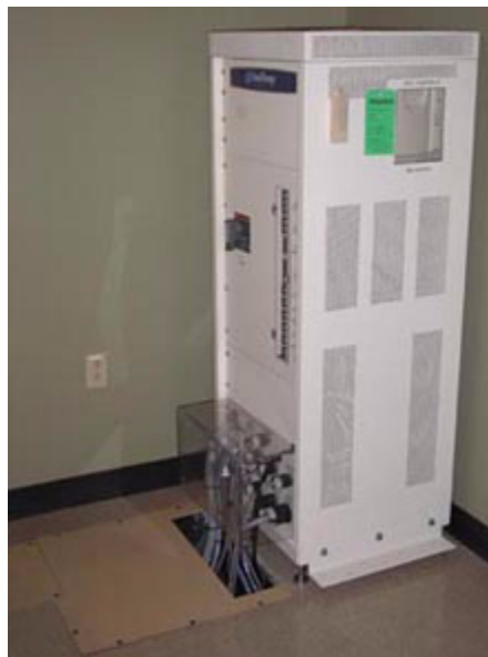
Figure 5-5: PDU with floor box cover plate.
