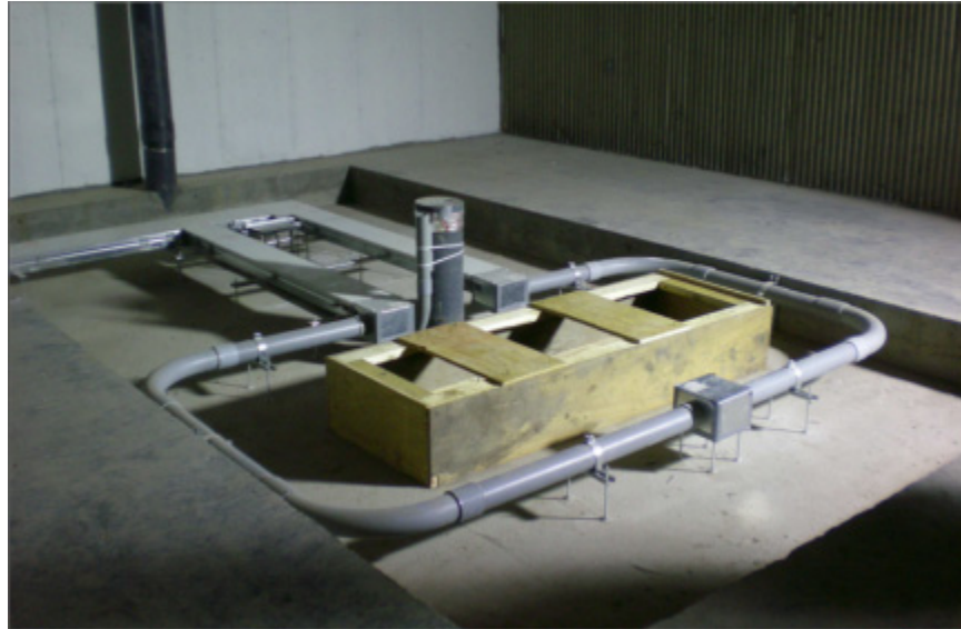
Figure 4-1: Gantry pit construction and utility routing before concrete pour.
