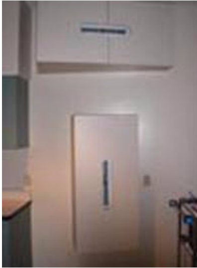
Figure 4-10: Surface-mounted lasers covered with cabinets.
