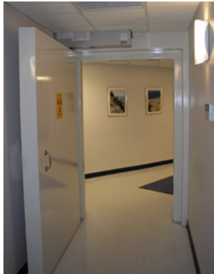
Figure 4-6: Standard Treatment Vault door.
