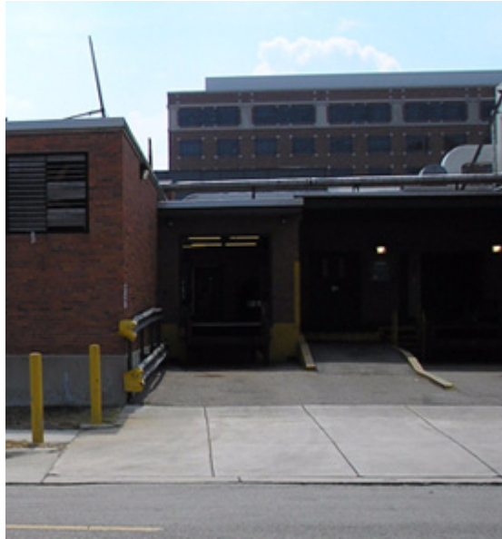
Figure 1-1: Facility loading dock.
