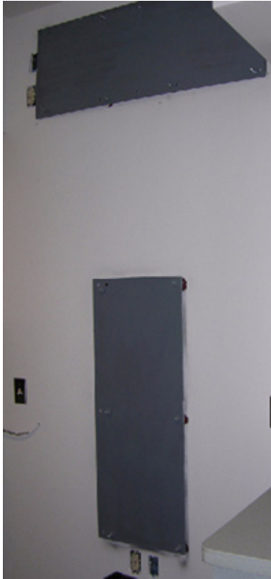
Figure 4-11: Dorado side laser plates mounted on the wall surface.
