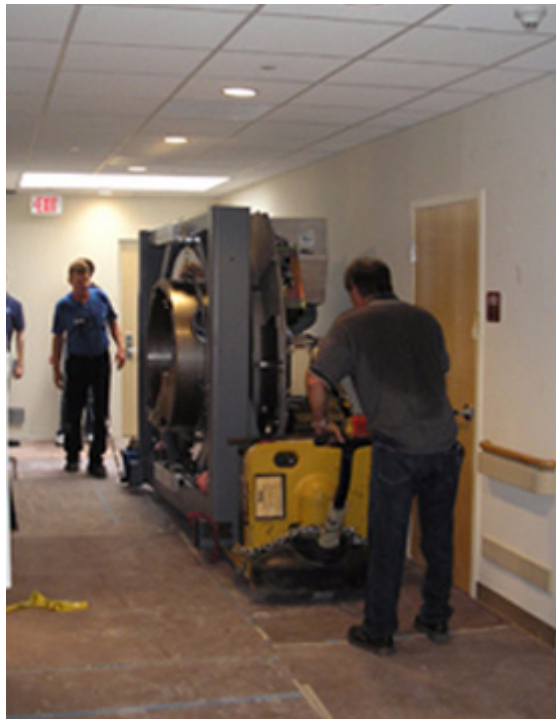
Figure 1-2: Gantry rolled through the facility hallway.
