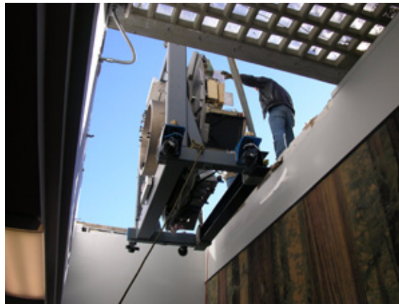
Figure 1-3: Gantry lowered by crane through a roof opening.
