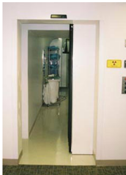
Figure 4-7: Sliding Treatment Vault door.
