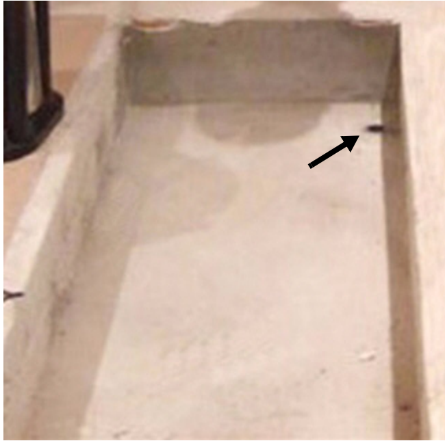
Figure 4-4: Gantry pit with floor drain.
